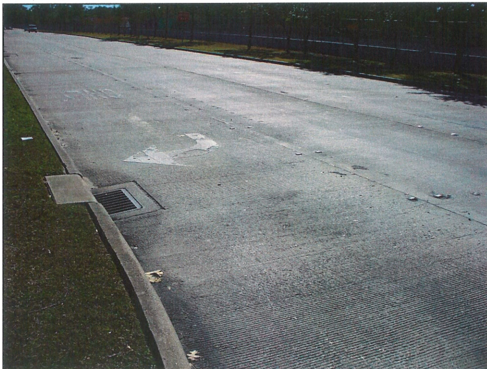
Photograph 12 - Memorial Drive @ Beltway 8 NSR Looking South
