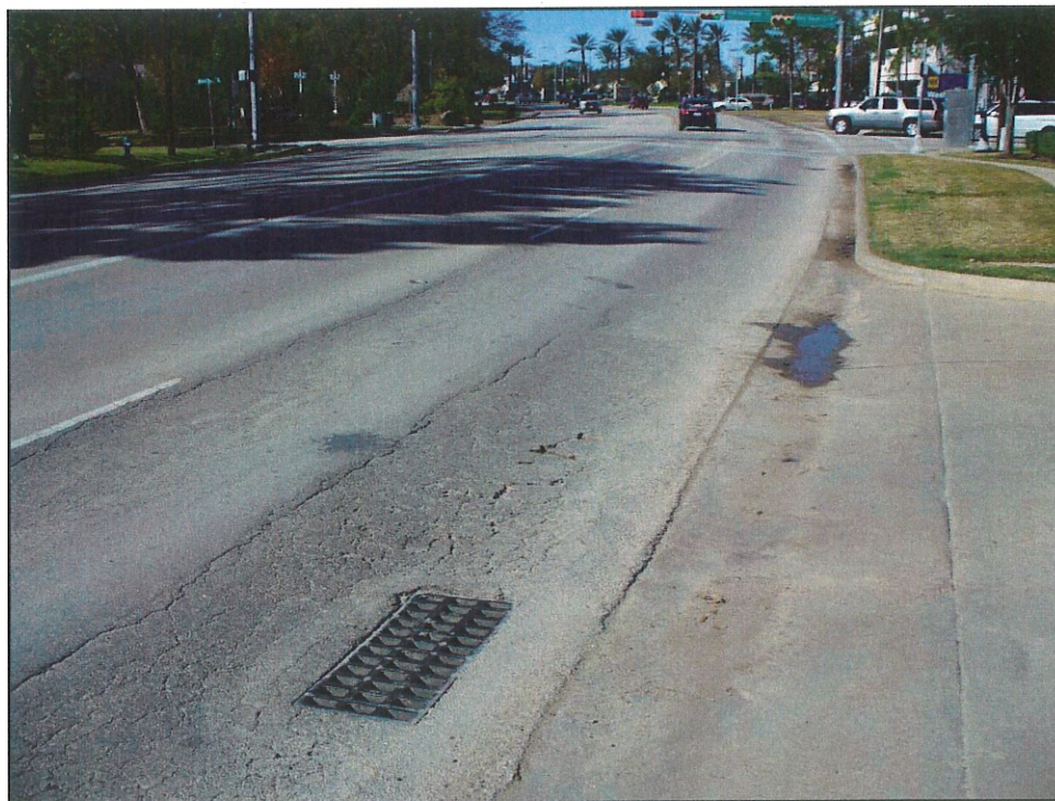
Photograph 4 - Memorial Drive @ West Bough Lane Looking West
