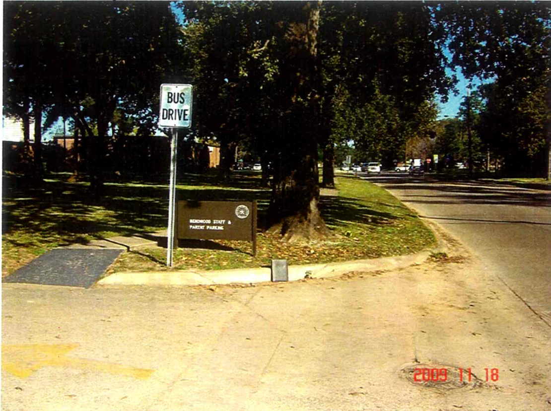
Figure 11: Yellow tape measure indicates 5' back of curb for sidewalk construction.
