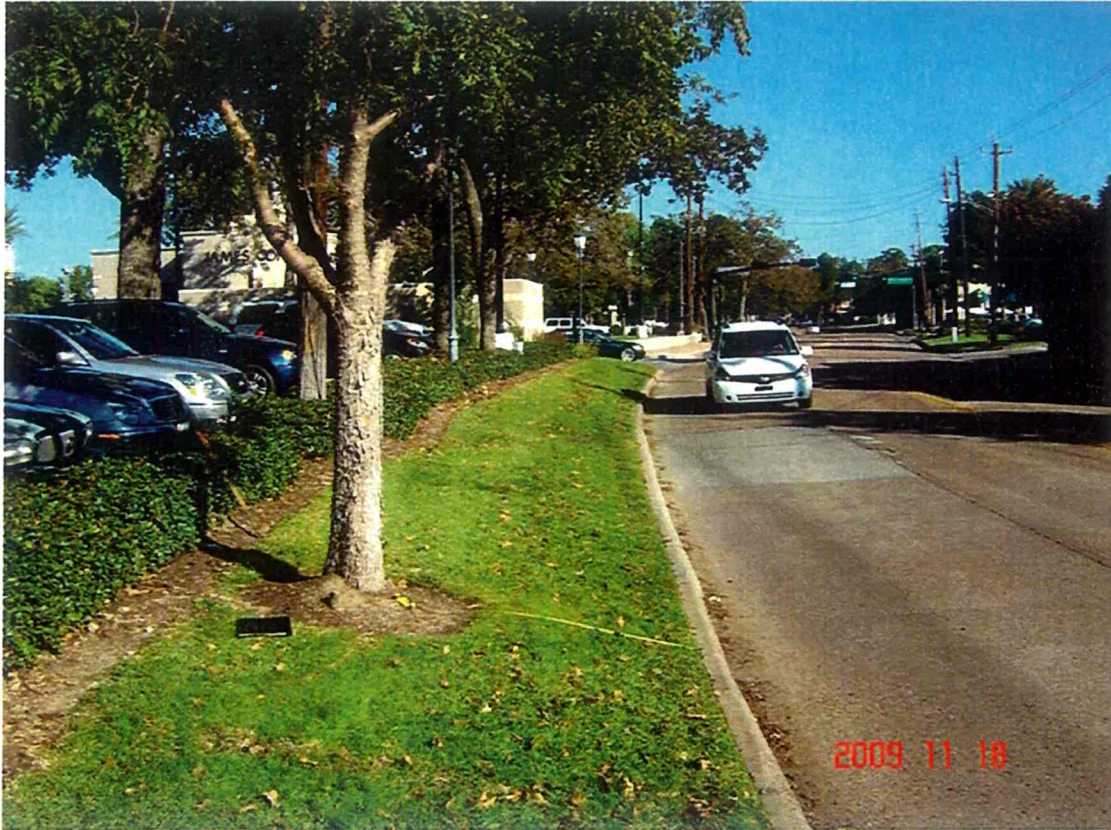
Figure 3: Yellow tape measure indicates location of 5' sidewalk immediately back of curb at tree 12.
