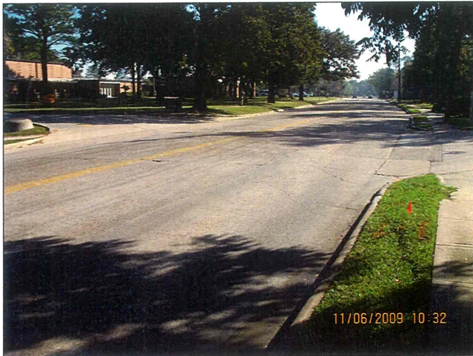
Figure D.3 – Kimberley Lane (Looking East)
