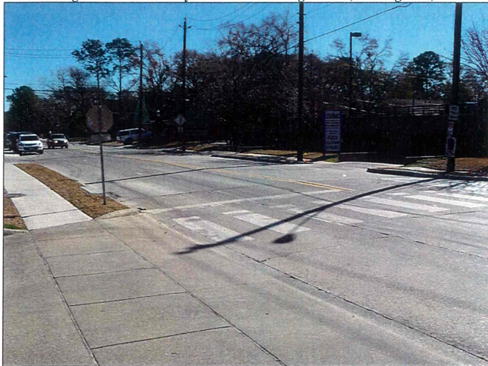
Figure 2.5 - Kimberley Lane @ West Bough Lane (Looking East)
