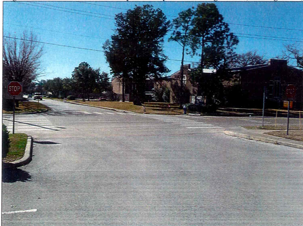
Figure 2.6 - Bendwood Elementary Driveway @ West Bough Lane (Looking South)
