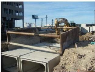
Storm sewer box culverts for storage and conveyance
