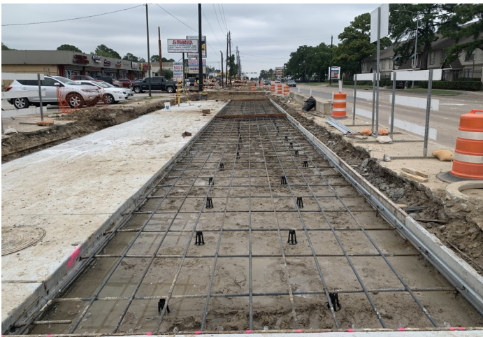
Forming and Rebar for pavement installation.
