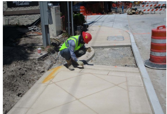
Installation of decorative sidewalks
