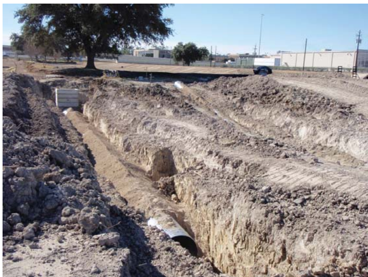
Phase II - 24" Back slope interceptor and 36" storm sewer connection at south end of basin.
