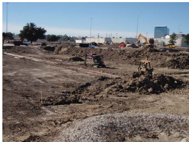
Phase II - Excavation continues while laying out pilot channels in bottom of basin.
