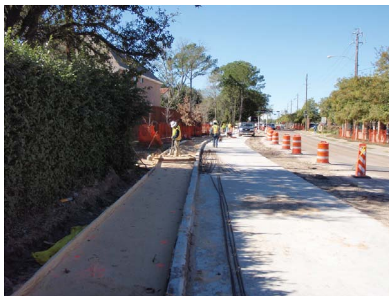
South lane paving complete and sidewalk in progress.
