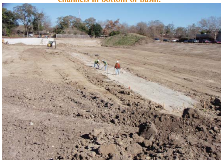
Phase II - Preparing base for pilot channel along east side of basin.
