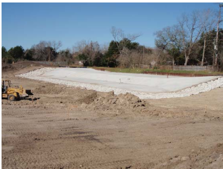
Phase II - Rip-rap placed along sides and base of weir structure.
