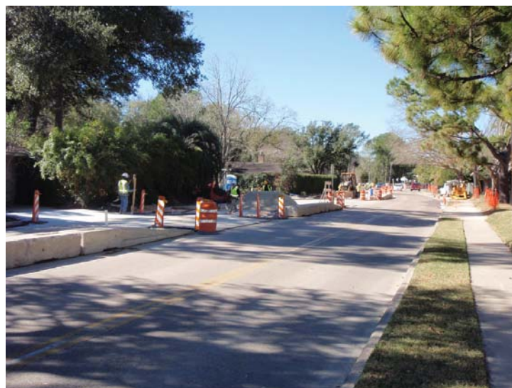
Completed residential driveway and south lane paving east of Barracuda
