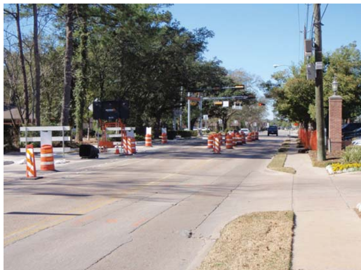
Traffic control relocated east of Memorial City Way, and intersection opened to traffic.
