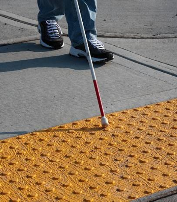
Truncated Dome Warning Devices
