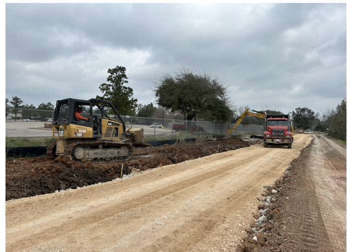
Basin Access Road
