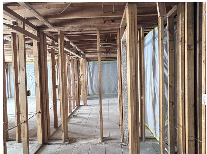
Abatement Work and Drywall Removal
