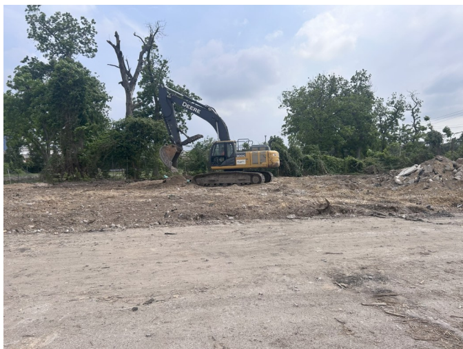
Concrete Foundation Removal
