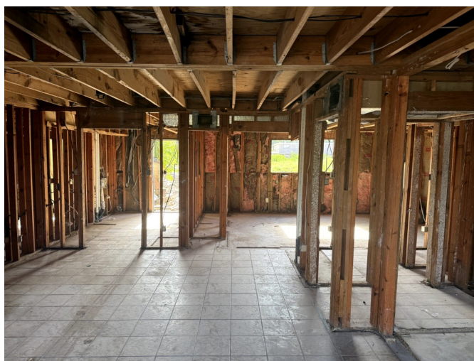
Drywall Removed—Building Ready to be Demolished
