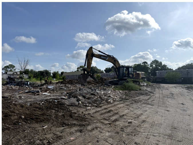
Concrete Foundation Removal
