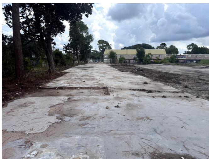
Remaining Concrete Foundation
