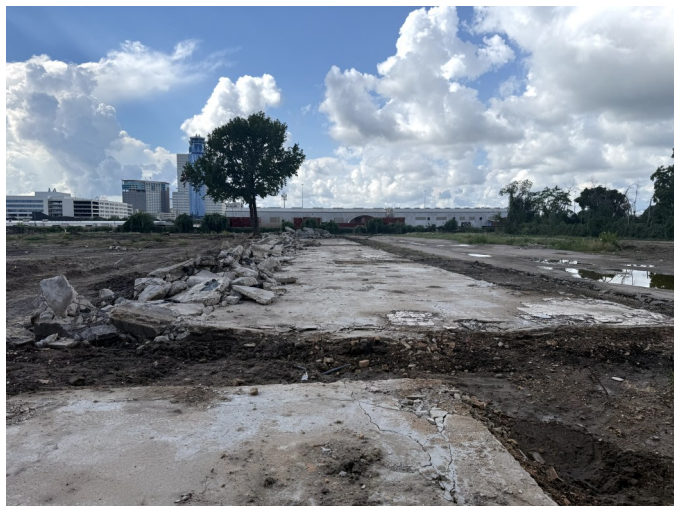
Concrete Foundation Removal
