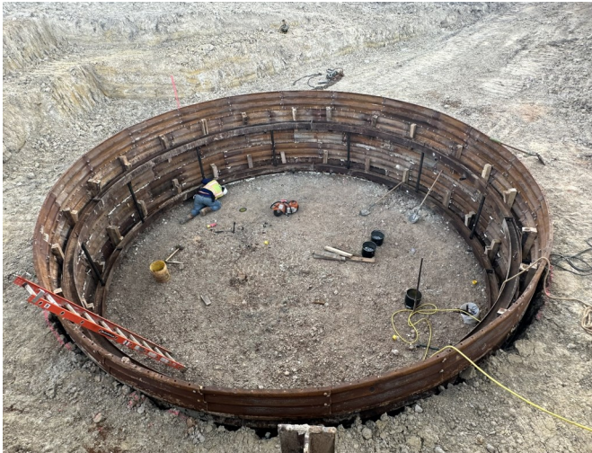
Liner Plate Shaft Installation for Wet Well
