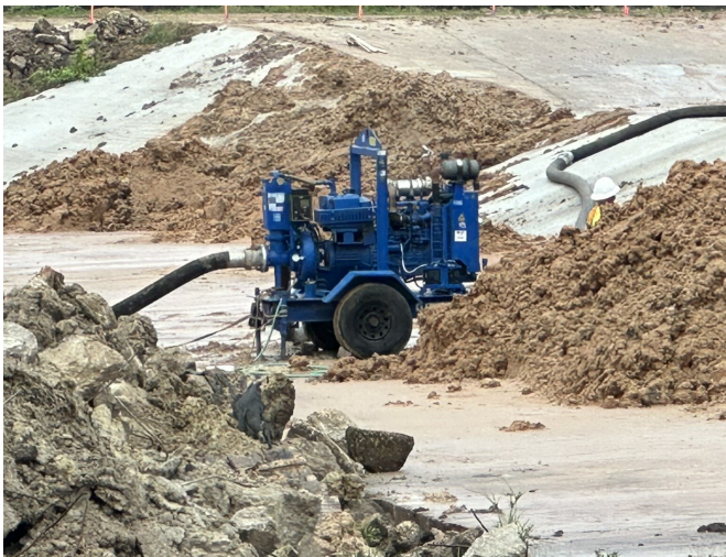
Pump for Ground Water Control
