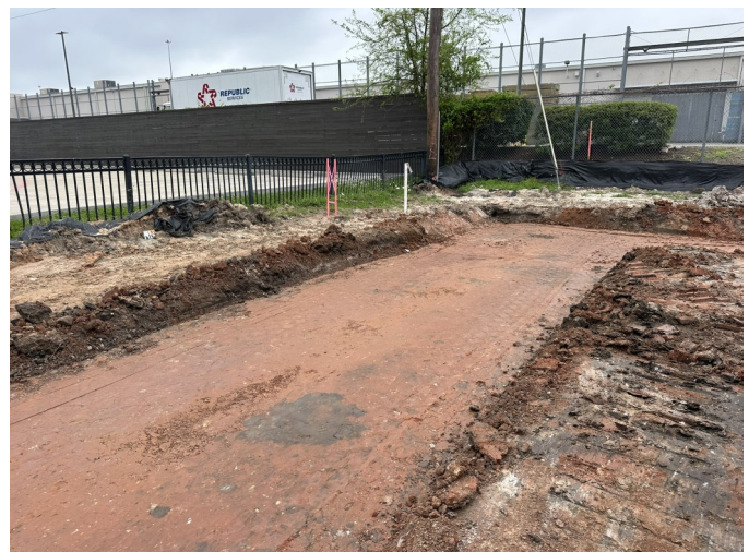
Slurry Wall Cap Installation
