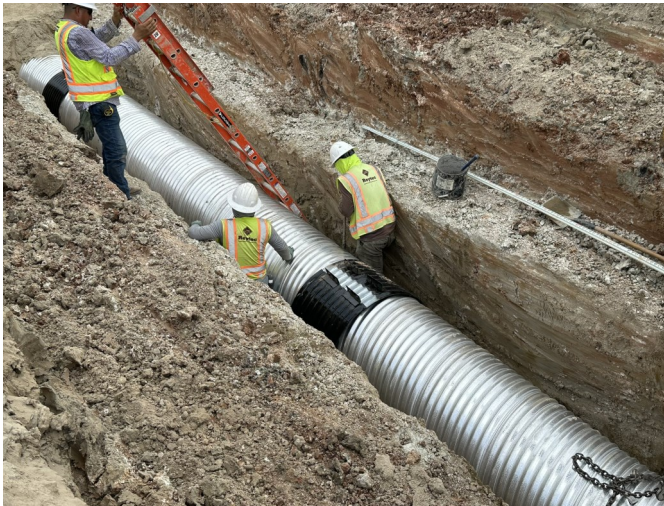
Storm Sewer Installation
