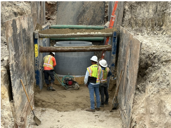
Manhole Installation
