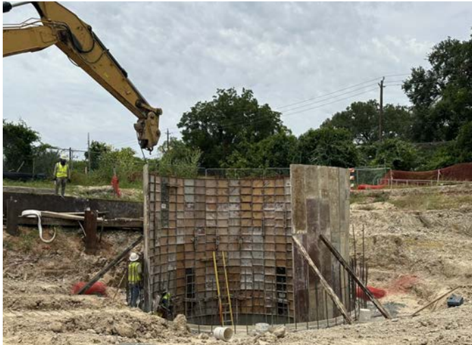
Formwork for Wet Well Top
