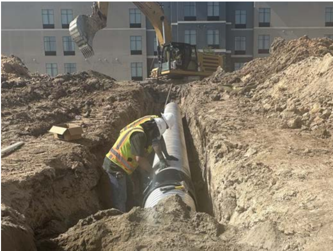
Backslope Interceptor Pipe Installation
