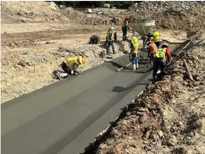
Concrete Pilot Channel
